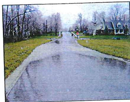
Looking northeast at Pebblebrook Place during January 5 th , 2005 storm event
